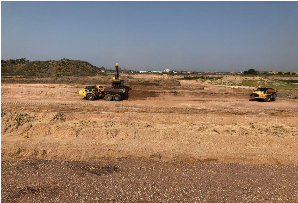
Extraction of the Core following completion of the Perimeter Extraction Keyway
